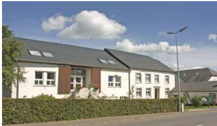
Figure 11. The 3rd CLESEN house is situated on a parcel that belonged to the property of the CLESEN ancestral house in the street to Ulflingen behind the museum.
